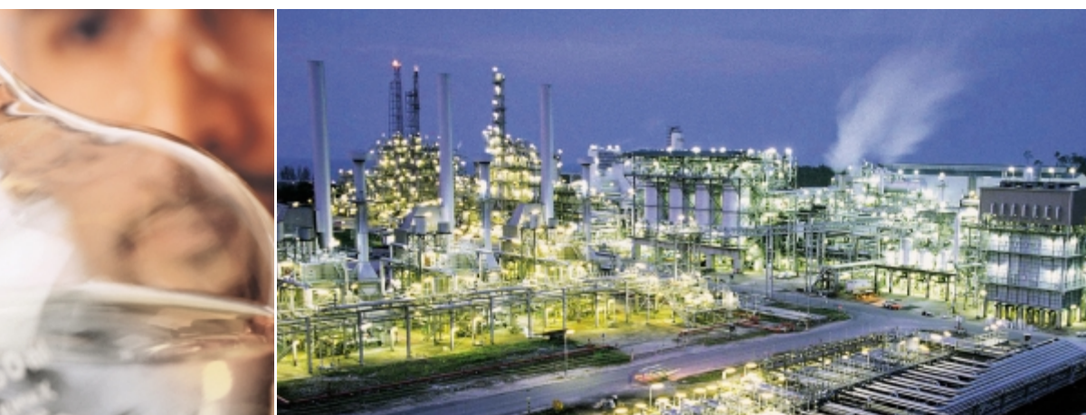
Producing high-purity SynFuel by Fischer-Tropsch synthesis since 1993: Shell's gas-to-liquid (GtL) plant in Bintulu, Malaysia (photo: Shell).
